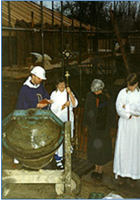
Topping Out December 1993
