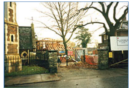
Building the hall
