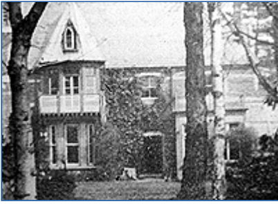
The original vicarage
